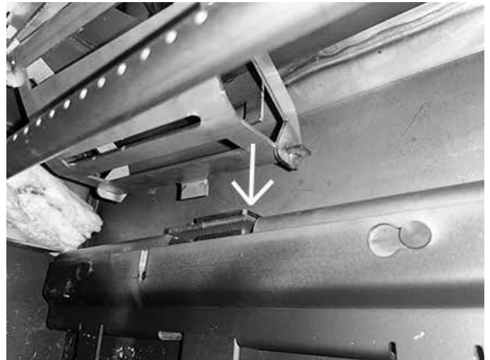
Figure 9: Remove Flue Gas Agitator
