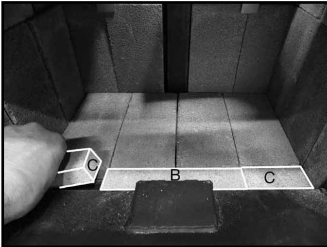
Figure 30: Narrow front bricks in place.
