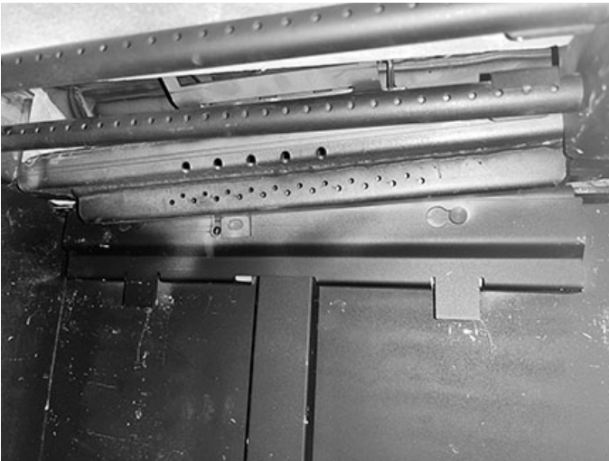
Figure 8: Remove rear baffle.
