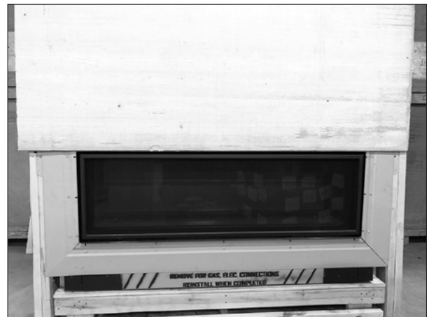
Figure 4.9, Installed Panels and Non-Combustible Material
