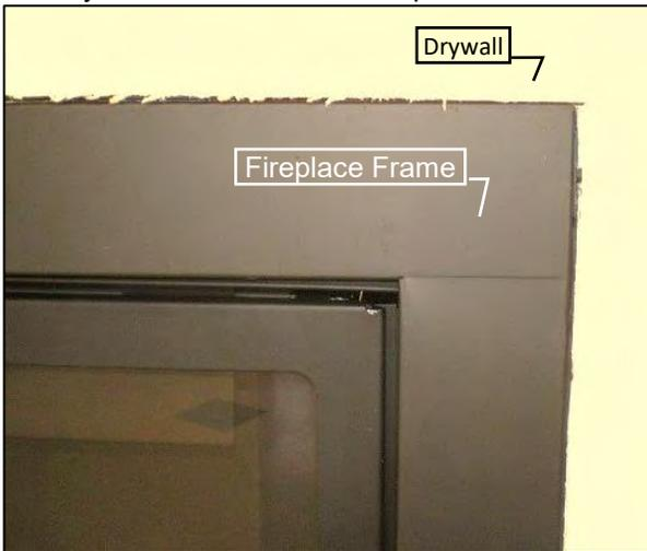
**Step 3:** Apply brick, tile, or other non-combustible material over fireplace face. **NOTE:** Leave clearance of 1-3/16" on top and 1-1/16" on sides and bottom to install and remove screen.
