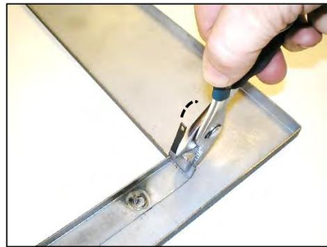
Place surround face down on protected surface. Bend Top Hook and Lower Mount Tab up 90° from surface.
