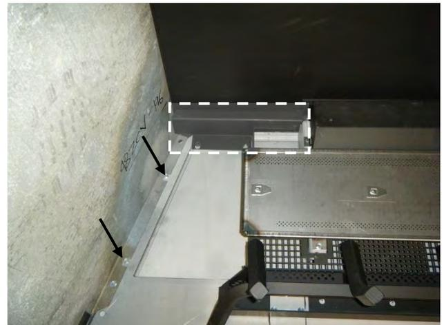
**Step Five:** Reinstall Liner Supports and Screws.
