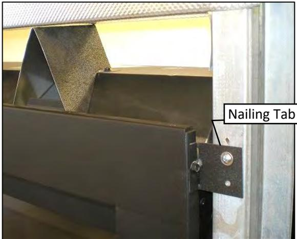
**Step 2:** Use Drywall to finish face of wall.
