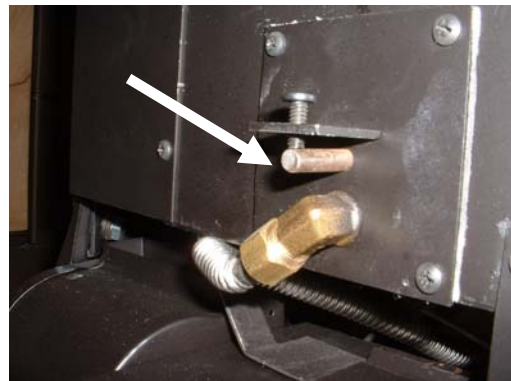
Photo 37 – Air Shutter Opened
