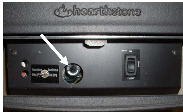
Photo 39 – ST Valve Output Control
