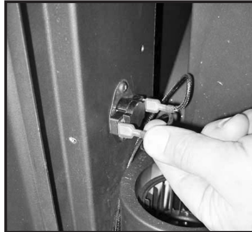
Figure 14: Disconnecting thermal switch.
