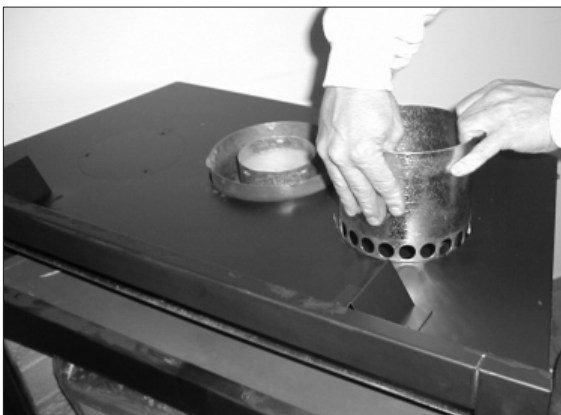
Figure 4.4, Duct Collar into Knockout
