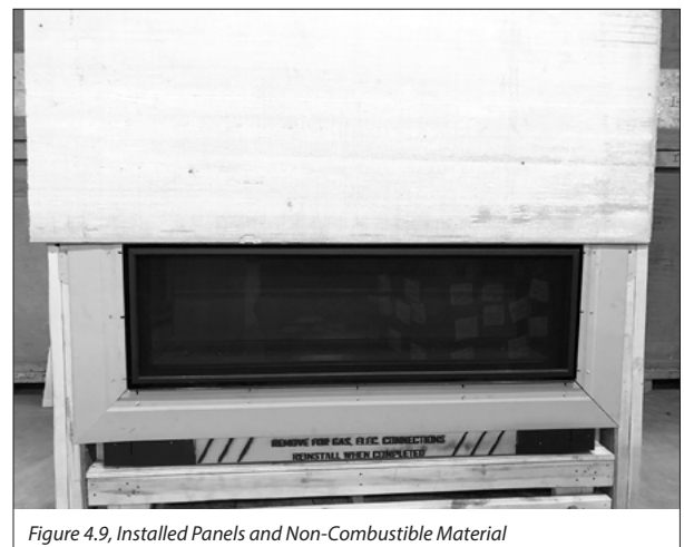
Figure 4.9, Installed Panels and Non-Combustible Material
